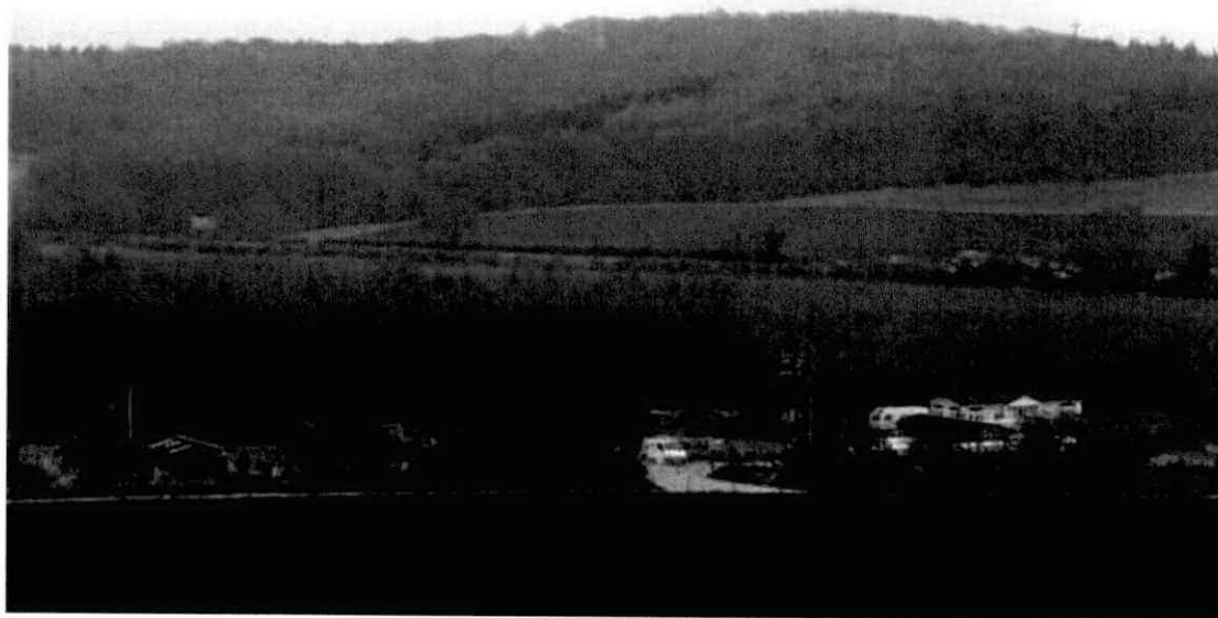
A view of the Traveller sites showing the visibility from the west
